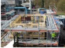
The builders make a wooden frame in the shape of the walls. This acts as a mould that the hempcrete can be poured into. All the gaps are filled.
