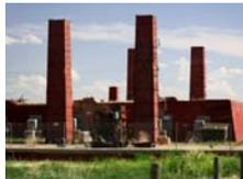
Lots of houses are built from bricks. Bricks are made from clay which is then baked in large, hot ovens. This uses a lot of energy. It can add a lot of carbon dioxide to the atmosphere. Using energy like this is adding to climate change.
